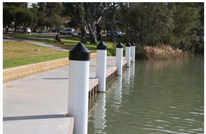
IR planks used on a Murray River landing at Mildura.
