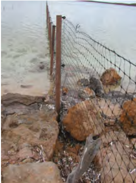
Close up view of the IR posts used in the Shark Bay, WA fencing site.
